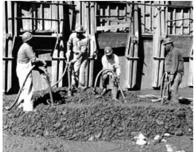
*Fig. 4.3—Consolidation of low-slump mass concrete placed by bucket.*
