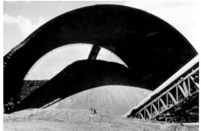
Fig. 4.4—Metal cover over drained fine aggregate stockpile to reduce heat absorption.
