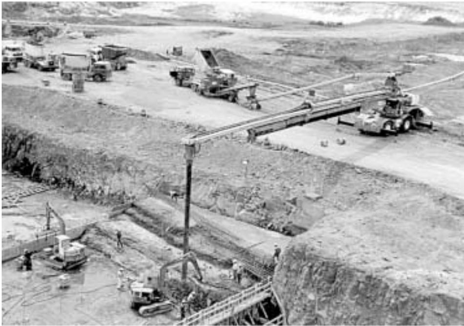
Fig. 4.2—Placement of mass concrete by conveyor belt.
