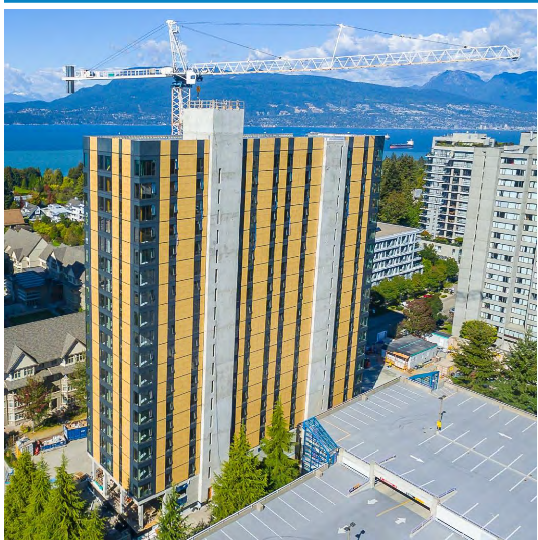
Figure 1: UBC Brock Commons Tallwood House. 6
